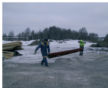
The Ultra Rib 2 pipes made from BorECO PP are lightweight and easy to handle.
