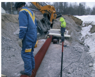
The twin wall BorECO PP sewage pipes made of Borealis material is the best choice for installation in icy conditions.
