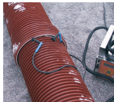
The electro fusion of the Ultra Rib 2 pipes made from BorECO PP is easy and fast and results in a leak-tight, high quality controllable seam, suitable for demanding ground water areas.
