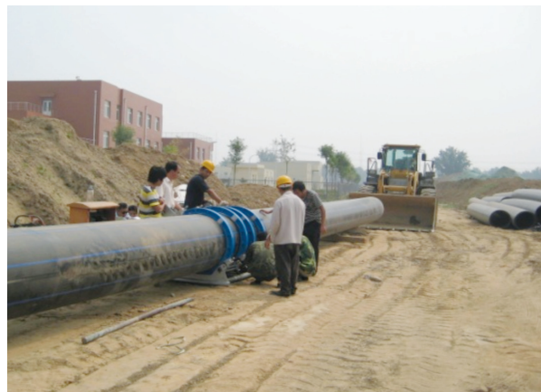
General view of the installation site
