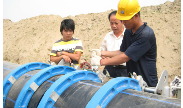
On-site butt fusion welding training
