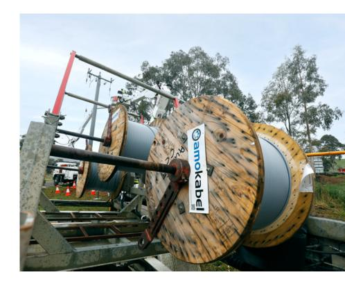
"The use of covered overhead line conductors has helped United Energy to manage the bushfire risk by providing a cost-effective retrofit solution for overhead line upgrades plus the potential to boost network reliability."
