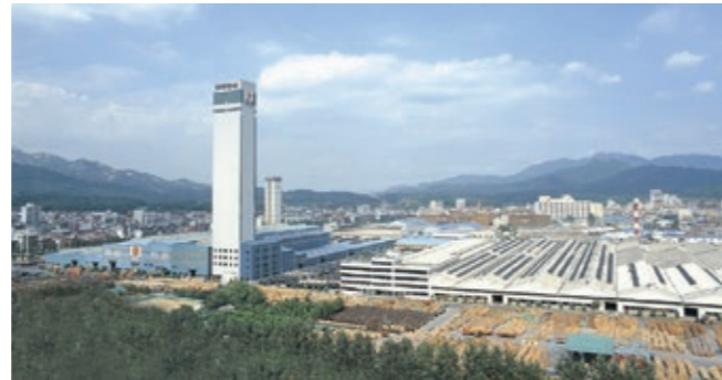
Taihand Electric Wire Co, Anyang plant
