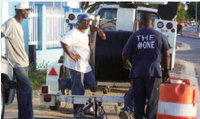
Picture 1. Installation of backbone at Bonaire
