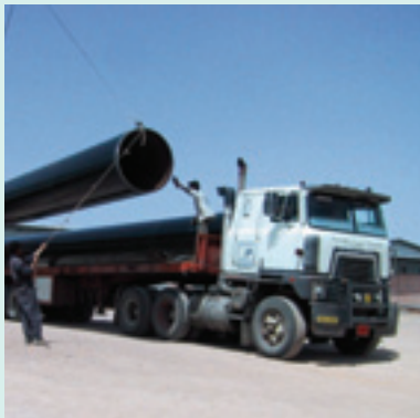
Transport of coated steel pipes
