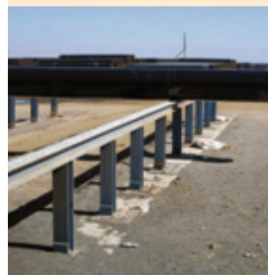
Pipe coating cooling rack
