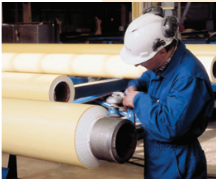
Borcoat pipes being prepared
