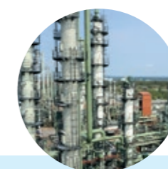
Acids and abrasive slurries at Hindustan Zinc, India
