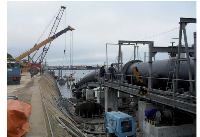
PE pipes being pushed into the water
